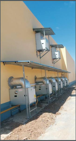
**Top Left Imagec:** Heat recovery ventilator installed outside the pigsty.
