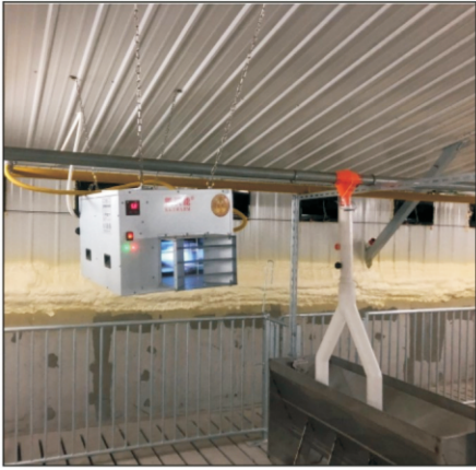
Aonong Group Dachuang Pig Farm
